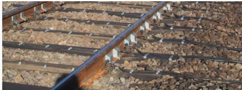
Sensor-based derailment detection system "Argos Derail"
